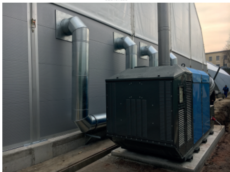
Fixinstallation Heizung (GAS)
