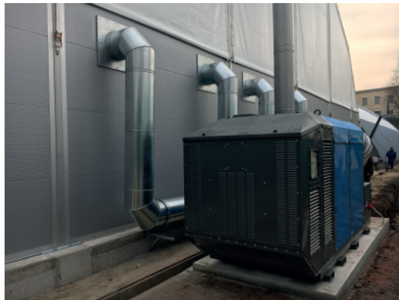
Fixinstallation Heizung (GAS)
